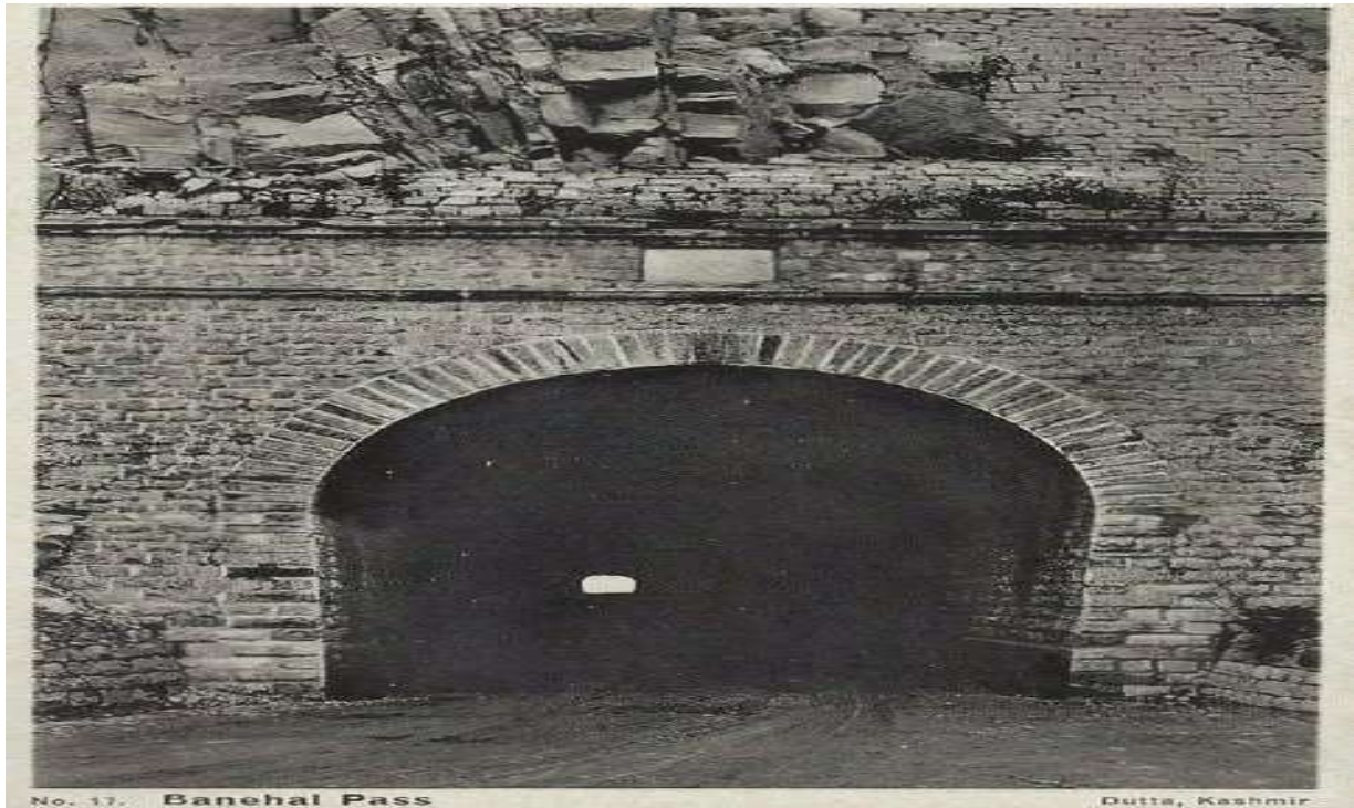
Fig.3: Old tunnel When it was operational in 1922
