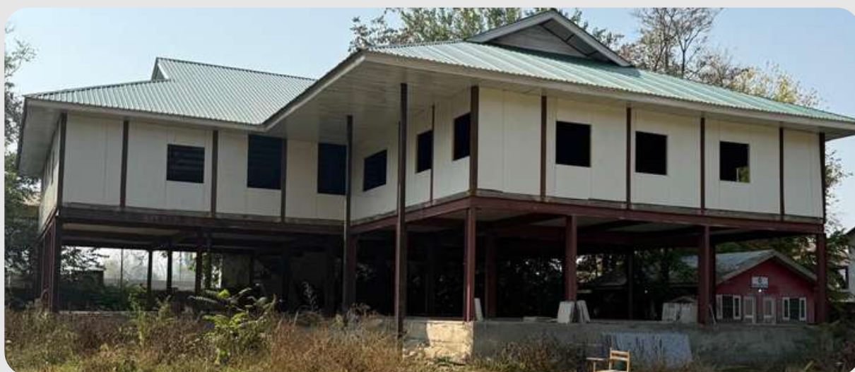
Under-construction Information Technology Hub
