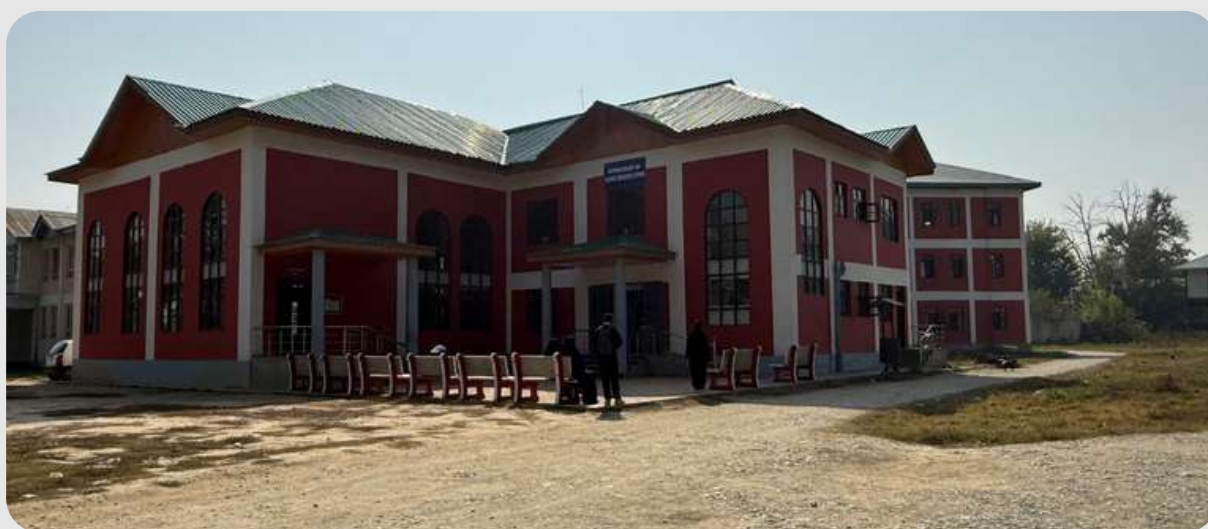
Newly Constructed Sports and Canteen Block
